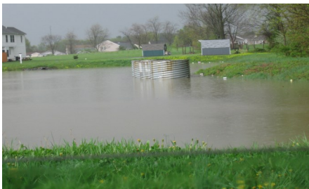
City staff will inspect detention ponds to make sure the facility is operating properly
