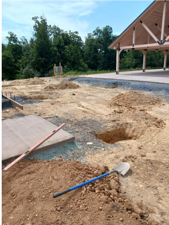
Shelter with concrete pad and work on tent anchors
