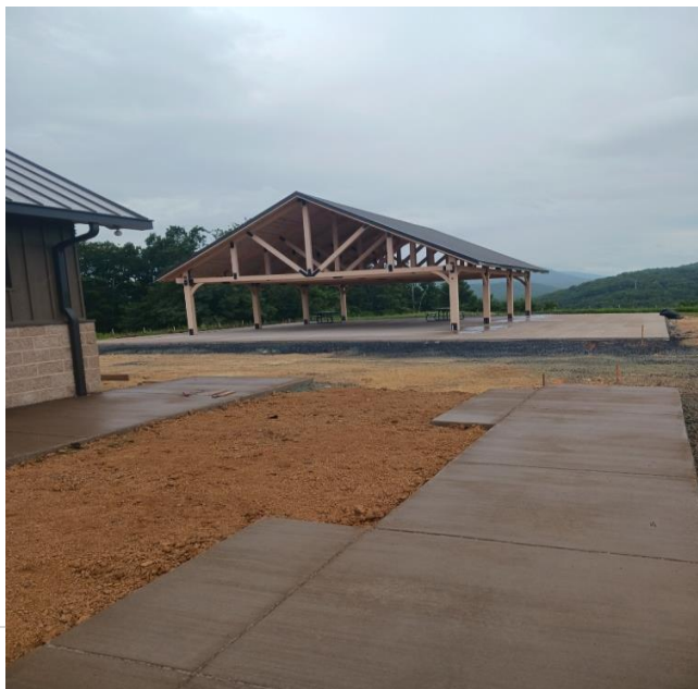
Shelter with concrete pad and sidewalk/bed area
